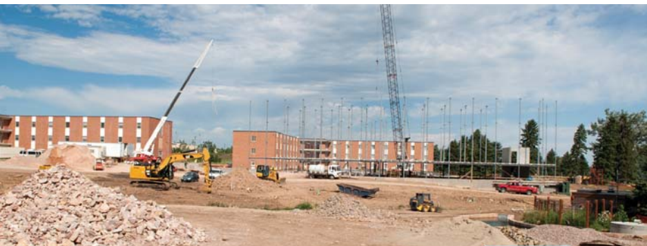
Construction is in progress on The Peaks, the student housing complex that will include Thomas, Hiedepriem and Crow Peak Halls.
