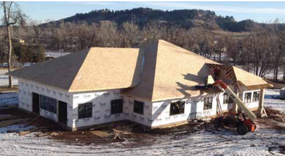
Construction began on the Joy (Proctor) Krautschun Alumni/Foundation Welcome Center in summer of 2013 and is expected to be completed this year.
